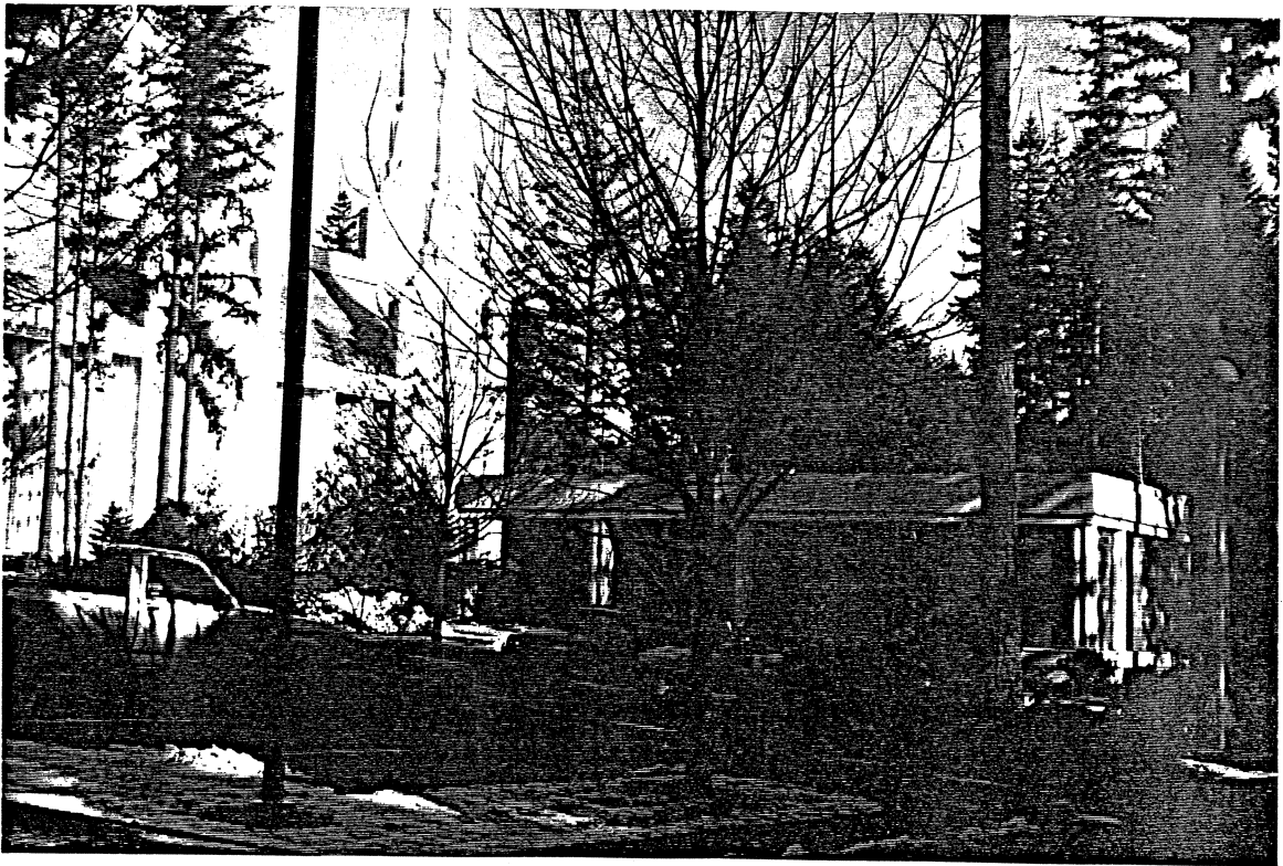
Wash building with tunnels connecting it to Mormon Temple.
